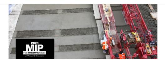
Originally designed to take on an exceedingly specific, labor intensive task and pave the areas between the raised rebar in the concrete plinths for light rail projects – Allen Engineering has reconfigured its new VLP 2424 to tackle a range of projects and paving application's, such as overhead bridge decks, light or heavy rail decks, roads, slabs on grade and ditch or channel pours.
