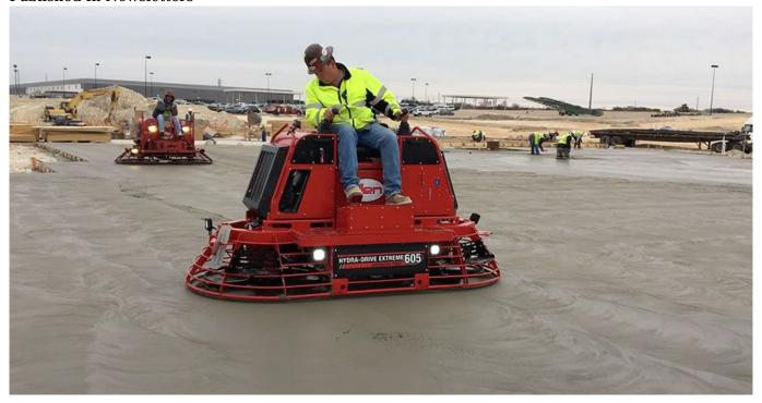
The HDX605 was designed with the high volume flatwork concrete contractor in mind. This new rider is not only fully hydraulic, but it also comes with cruise control, digital readouts for accurate fuel levels and diagnostics, and a large 13 gallon fuel tank for longer run times. It is also equipped with powerful pumps that help maintain excellent torque even at high rotor speeds. This makes the machine excellent for panning or finishing operations.
