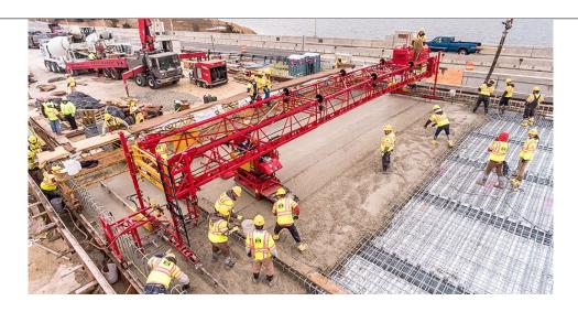
Increase your productivity and efficiency on jobs with this transverse roller tube paver. The machine advances automatically after each pass of the paving carriage and meters, consolidates, screeds to grade, smooths & textures the concrete. This paver offers significant time and labor savings.
