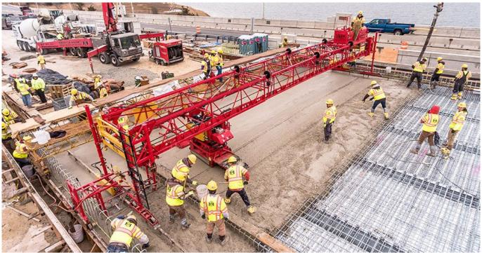
Increase your productivity and efficiency on jobs with this transverse roller tube paver. The machine advances automatically after each pass of the paving carriage and meters, consolidates, screeds to grade, smooths & textures the concrete. This paver offers significant time and labor savings.
