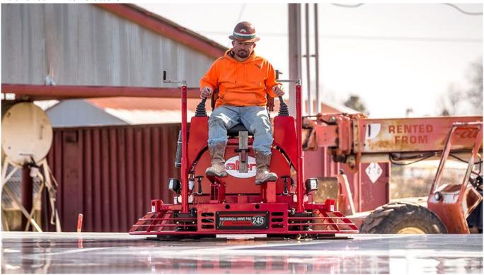
Increase your efficiency on jobs with this compact rider. This machine packs all the ergonomics, features and durability found in our larger riders in a smaller package that is perfect for quickly finishing pours that would normally requires several walk-behind trowels.
