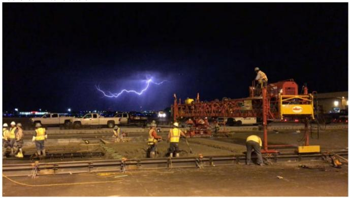
Allen Bridge Deck Finishers or transverse roller tube pavers have become a more viable option for concrete paving contractors due to the machines' ability to consolidate, screed & finish various types of concrete pavement projects.
