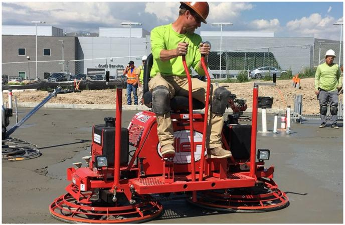
In May of 2017, Scoffield Construction Inc., was tasked with laying a concrete floor for the new Chick-fil-A in Lehi, UT. This pour had large amounts of piping and utility outlets making the job site tricky for a standard riding trowel.
