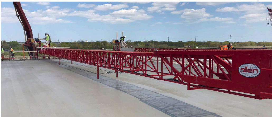
The cable tension kit and our telescoping section is being used on the WB2434.
