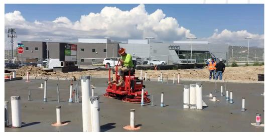
guard rings, allows you to run along the edges of walls, around columns and pipes-for a close, clean finish every time. This exclusive Allen rider allows you to edge within 5/16" of the edge of a wall, eliminating the need to hand finish those areas. This trowel features a stretched frame for improved productivity and operator comfort.
